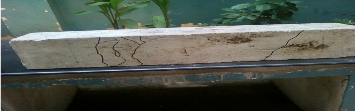
Figure 5(b): Flexure cum Shear failure pattern of S.S.R.C beam
